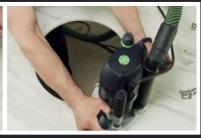
2. Drill the corners of the template, then use a milling machine at a 45 degree angle. Make holes 9mm wide and 10mm deep.
